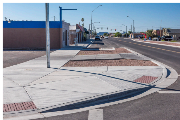
Coolidge Avenue Reconstruction Project
