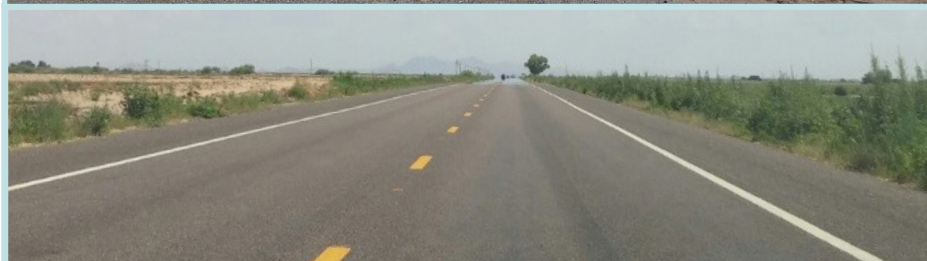
Example of a roadway with good pavement condition
